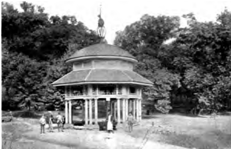
PLEASANT BEING THE INDIANA WHEELBAR, ON THE MICHIGAN RAIL
